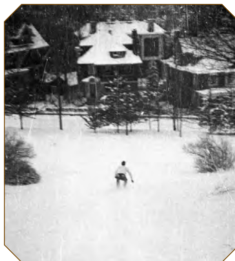
Sküing down the hill from the chapter house to Stewart Avenue, Jan. 1939
